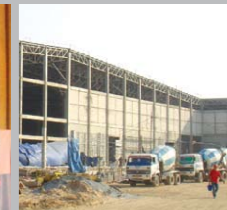
"Built-to-suit" warehouse under construction.
