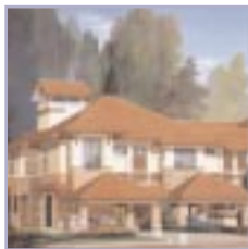
Double Storey Terrace House, Aman Suria Damansara
